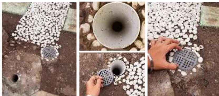
Gambar 5. Lubang Resapan Air Hujan Biopori
